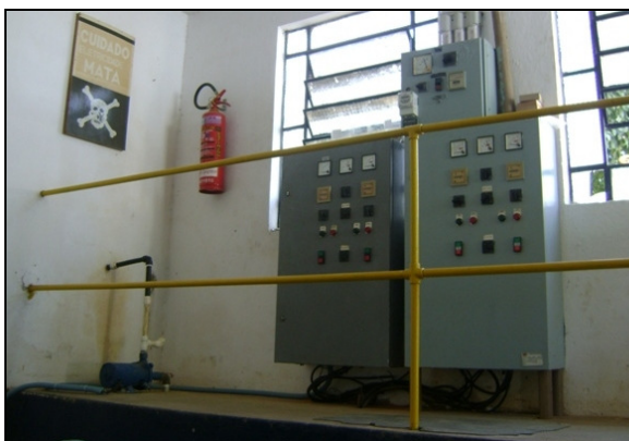
Foto 23 – Quadro de comando das EEPAs-02, EEPAs-03, EEPAs-04, EEPT-01 e EEAT-01.
