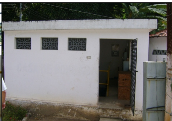
Foto 24 – Prédio de abrigo das EEPAs-02, EEPAs-03, EEPAs-04, EEPT-01 e EEAT-01.
