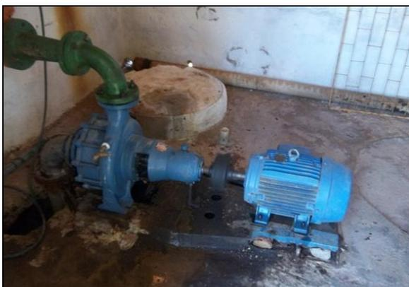
**Foto 3** – Conjunto moto-bomba do PA-01.
